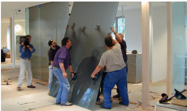
Installation of transparent glass panels
